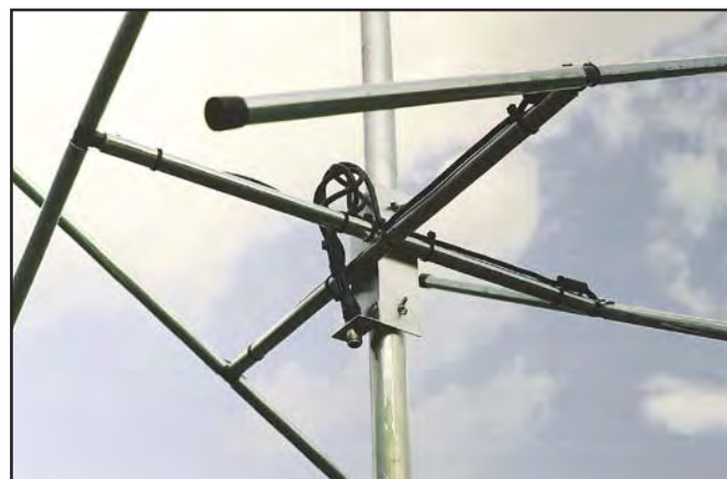
Figure 3 — View of cross booms mounted to mast.
